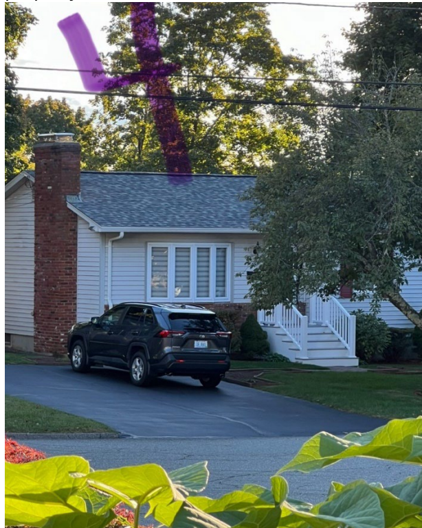
PHOTO 4. View of neighbor showing siding
