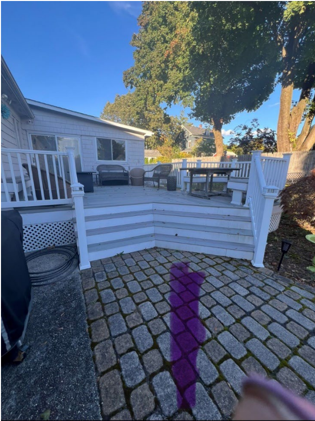
PHOTO 1. Existing vinyl deck attached to house
